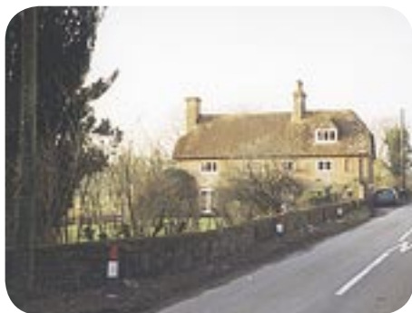
Island Mill from the south
