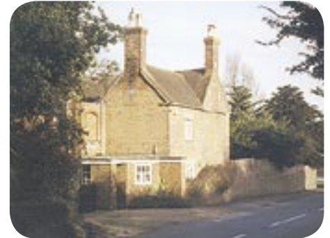
Hurstbourne Priors House and brick boundary wall
