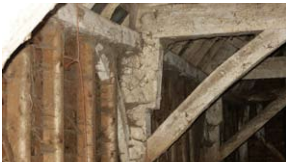
Above left: Jowls to post openings Above right: Blocked window
