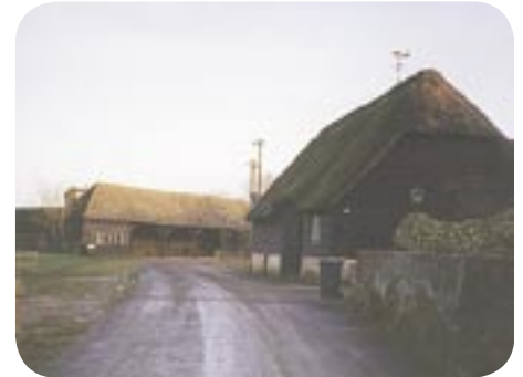
Listed barns at Manor Farm
