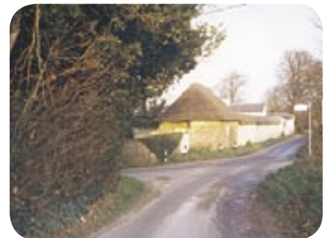
Cob and thatch boundary walls to the Manor House
