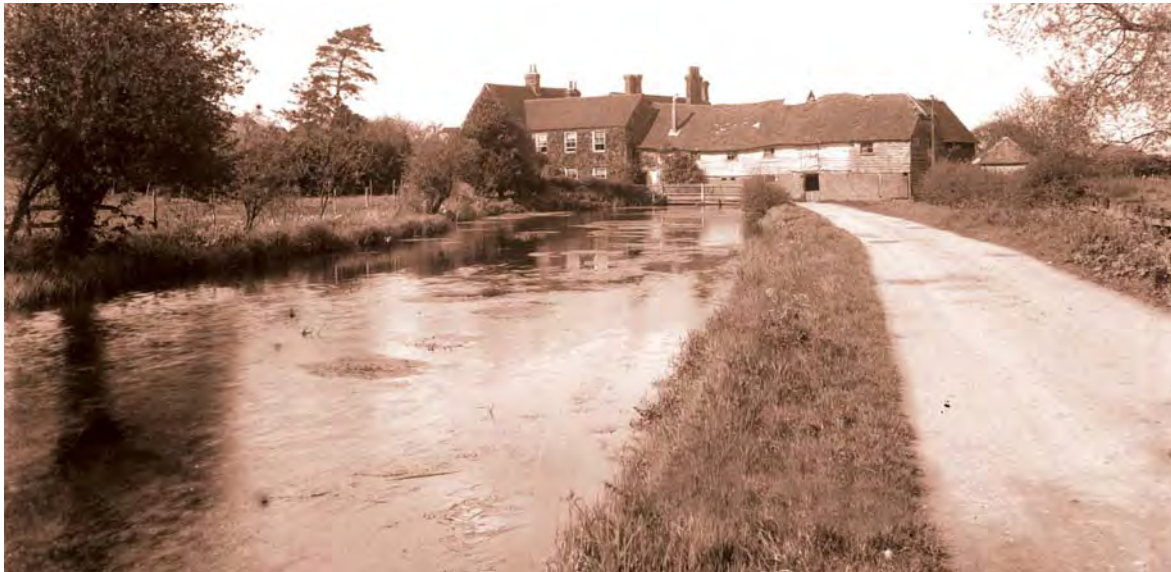
▲ Barton's Mill viewed from the railway viaduct; photo circa 1920's
