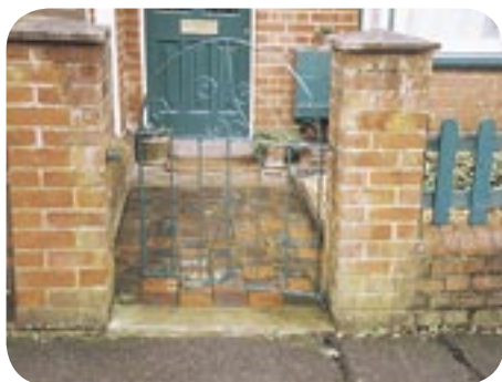
Original quarry tiles, Alexandra Road
