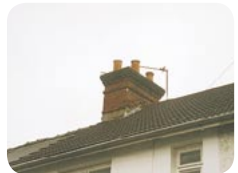
Chimney detail, Alexandra Road
