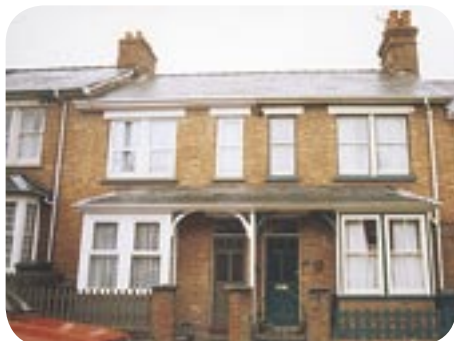
Combined porch and bay roofs, Alexandra Road
