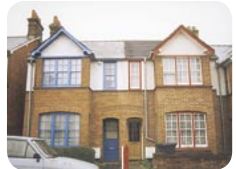
Two-storey bays at Alexandra Road
