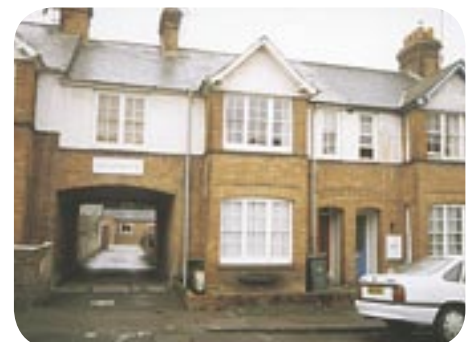
Passageway at Alexandra Road
