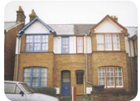
Two-storey bays at Alexandra Road
