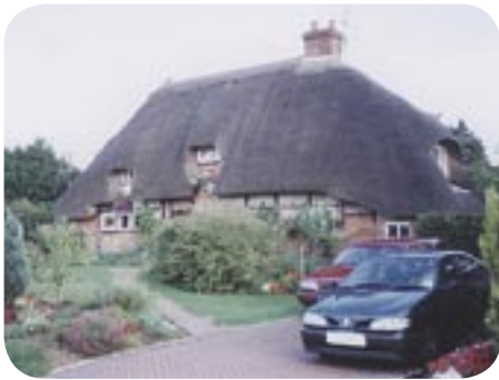
The Nook, Up Street. Timber-frame and thatch, dating from 1424 with 17th and 18th century alterations.
