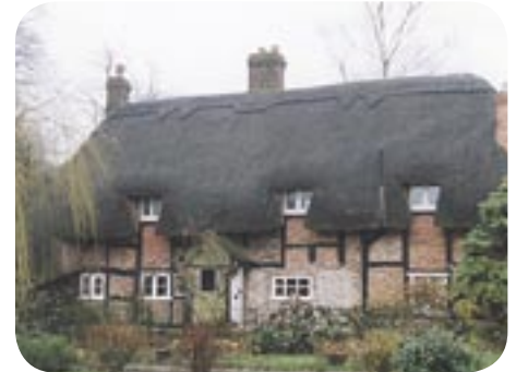
Well House, Down Street 17th century timber-frame with brickwork
