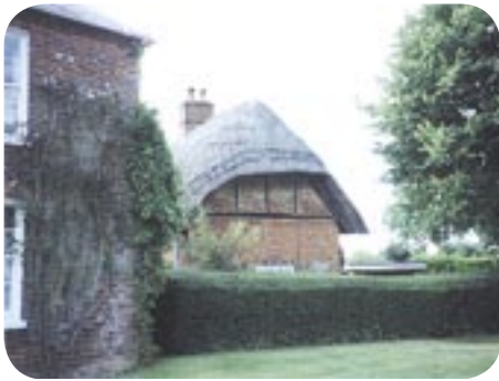
18th century brick timber-frame and thatch hip elevation of The Cottage, Down Street
