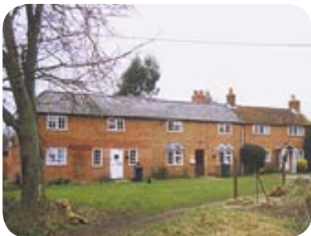
Former Forge Cottages
