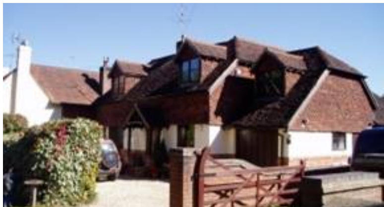
A new house built with old materials
