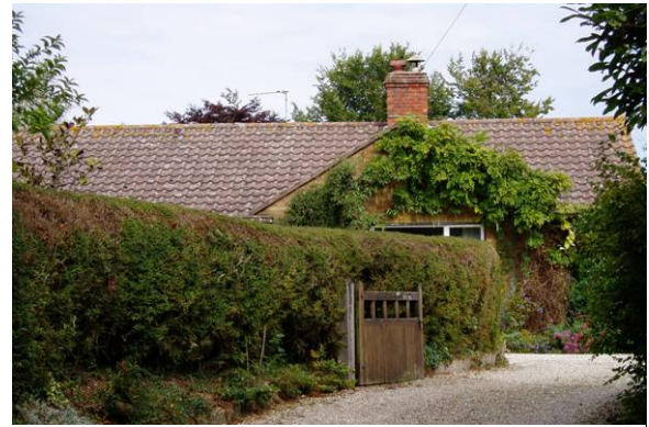
Detached Bungalow in Woods Lane
