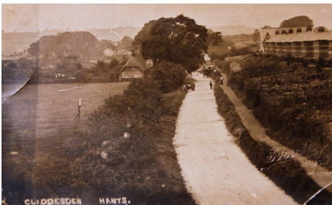
Looking South West along Farleigh Road, Southlea Cottages to the right, Southlea Meadow to the left, flooded
