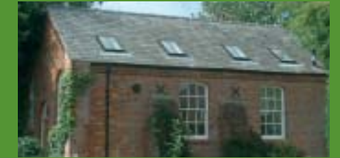
Rooflights avoid dominating a building of historical interest – Old Chapel, Down Street.
