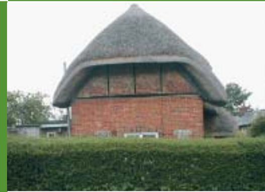
Hipped roof above timber frame – The Cottage, Down Street.
