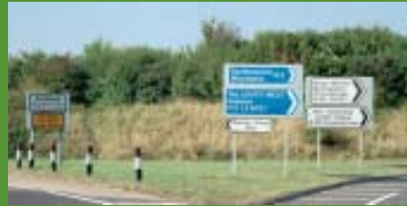
Confusing signs at junction 7 of the M3.
