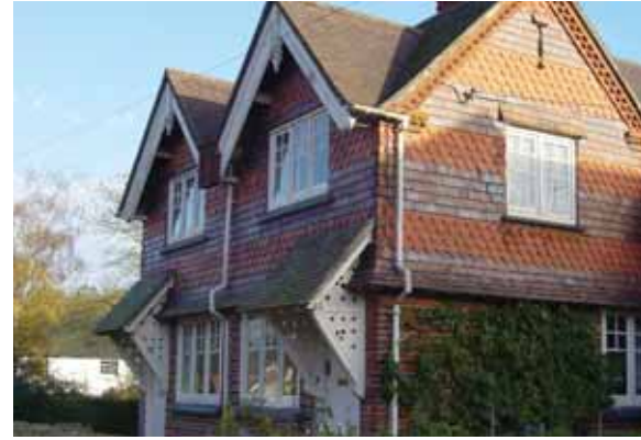
Victoria Cottages, East End. Decorative and plain Hollington tile in contrasting bands of colour. Hollington brick in English bond to give contrasting stripes of colour. Variable roof geometry, chimneys. Tiled canopy over door
