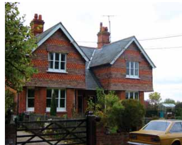
New Villa, Gore End. Slate roof, substantial chimney stacks. Decorative and plain hanging tile in bands
