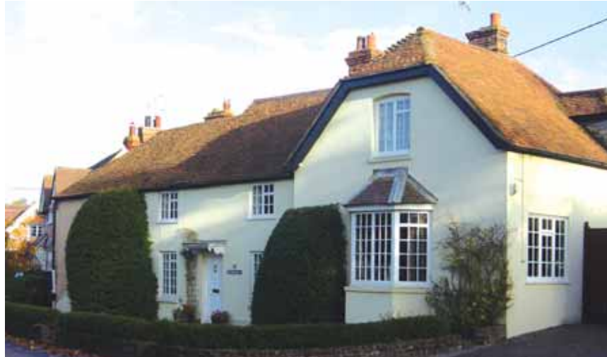
The Old Sun Inn, East End (early C19). Variable roof geometry, hipped, half-hipped dormer windows. Low height to eaves and ridge. Slate roof to rear. Painted render walls. Canopy on brackets over door. Windows in reveals
