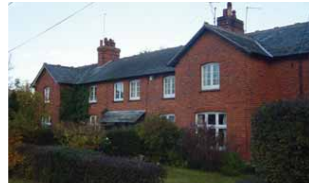
Wellington Cottages, Ball Hill. Hedge to road frontage. Terraced houses. Chimneys, low height to ridge and eaves. Windows in reveals. Cantilvered roof over doors
