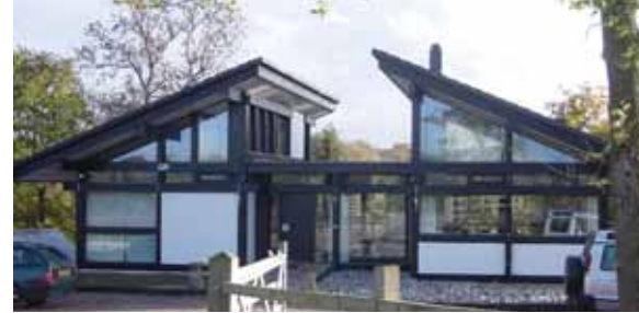
Northways, East Woodhay (2002/3). A Huf House. Glass and timber frame over concrete substructure.
