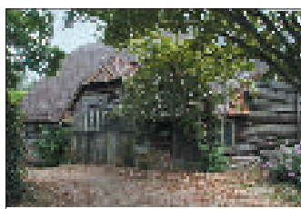
Barn at East Oakley House
