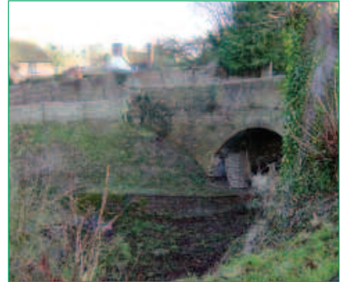
Basingstoke Canal at Basing House bridge
