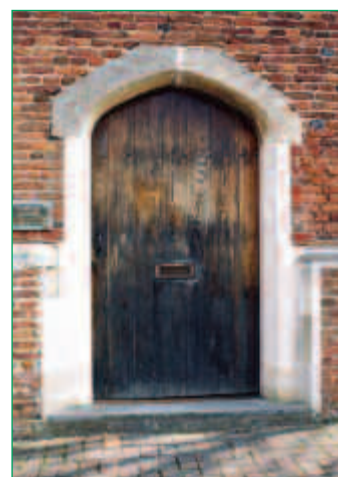
Doorway of doctor's surgery behind Lychpit Hall
