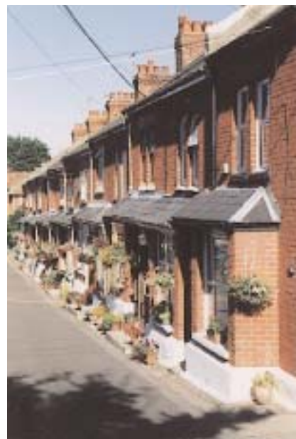
Right: Battens Avenue. The road separates the dwellings from their front plots
