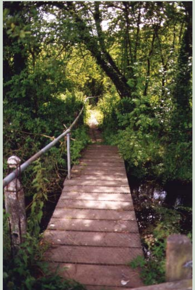
Trip-trap bridge on footpath north
