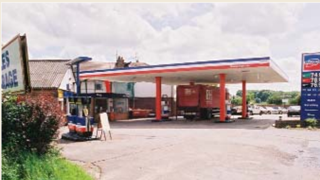
Gales Garage, Aldermaston Road
