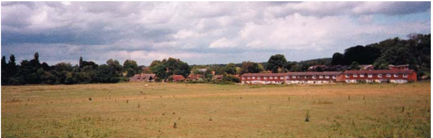
View from Sherborne Road towards the Vidlers Farm flats
