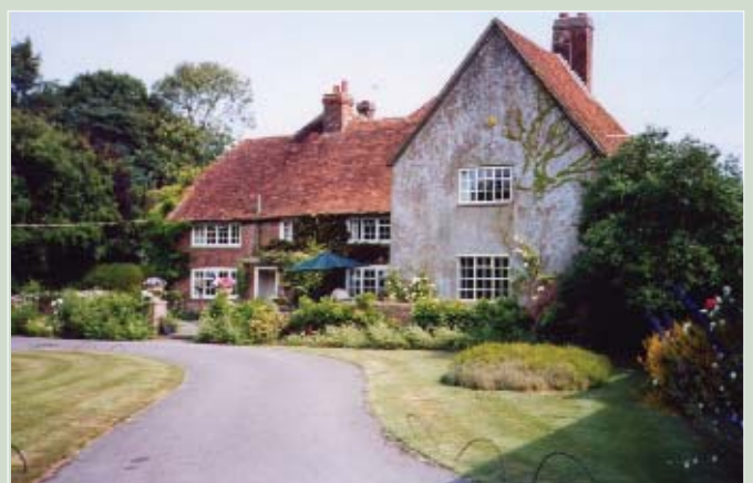
Cranes Farm House
