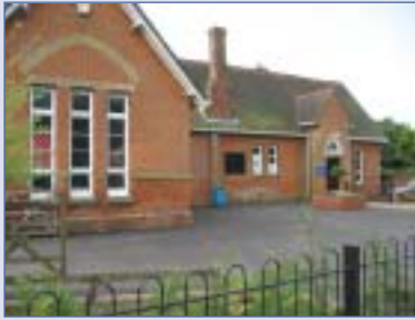
Tadley School with its Victorian Facade
