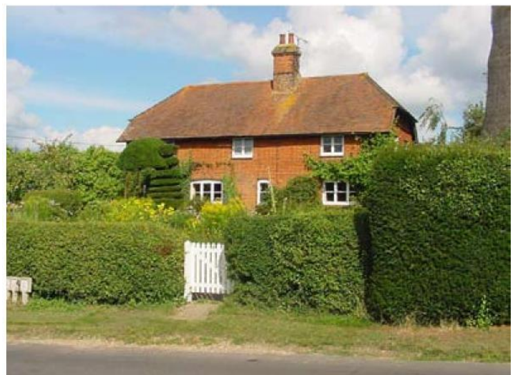
Half-hipped clay tile roof, Old Basing
