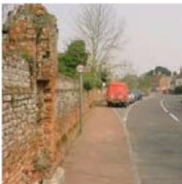
Old Basing. Brick boundary wall and buildings.
