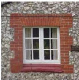
North Waltham. Flint with red brick dressing around a casement window.
