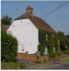
Highclere. Half-hipped roof with red clay tiles.
