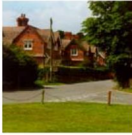
East End. Vertical clay tile hangings.
