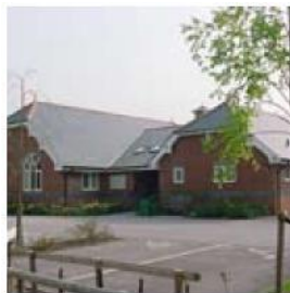
Cliddesden. The new village hall has picked up on local design details.
