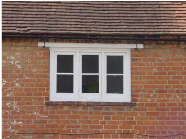
A typical casement window in a vernacular red brick and clay tile house, Old Basing
