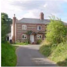
Egbury. Bands of brick and flint are a feature of many vernacular buildings.
