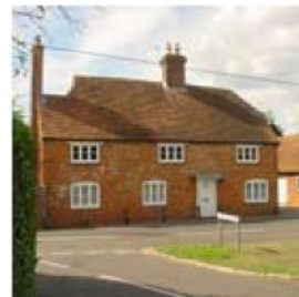
Old Basing. Many of the traditional buildings have first floor casement windows immediately beneath the eaves.
