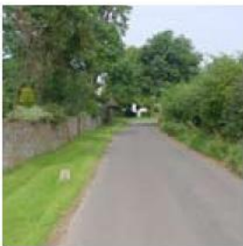
Steventon. Flint and brick boundary wall.
