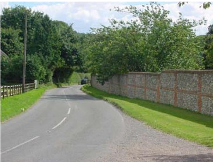
Flint and brick have frequently been used in boundary walls such as this one in Nutley
