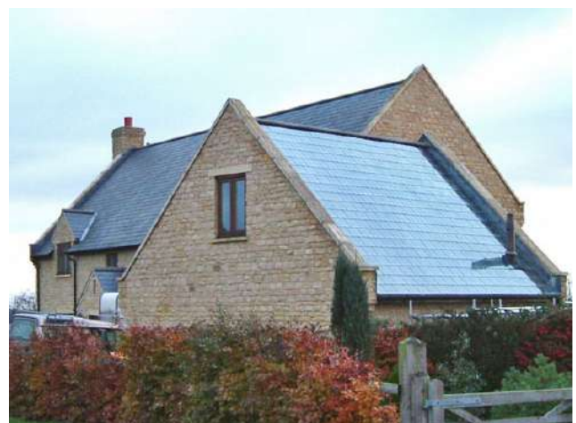
Figure 52: Positive example of implementing solar panels since the design stage.
