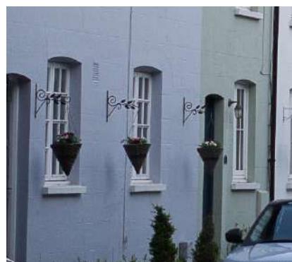
Figure 33: Iron hanging planters on the front building facade.
