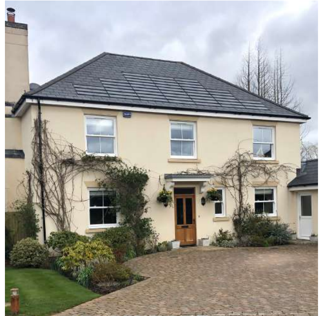
Figure 51: Use of shingle-like solar panels on a slate roof, with the design and colour of the solar panels matching those of the adjacent slate tiles.
