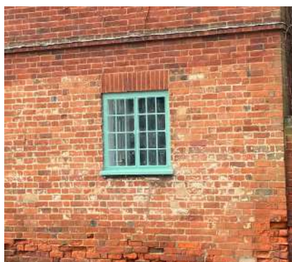
Figure 26: Recessed painted wooden window frame with vertical brick header.
