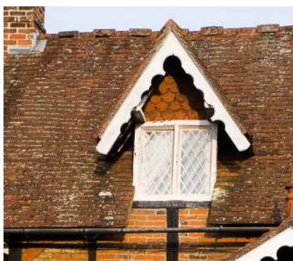
Figure 25: Pitched roof dormer with decorative, painted, wooden barge board.
