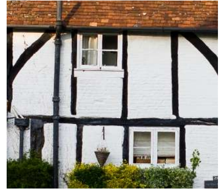
Figure 19: White painted brick and timber framing.
