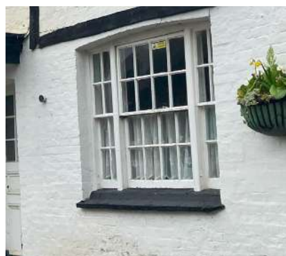
Figure 27: Recessed sash window with white, wooden frame.
